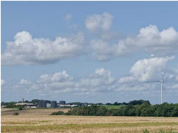
3D visualization of Electrochaea's bio-methanation plant at the Rybjerg Biogas plant_ ©Electrochaea
